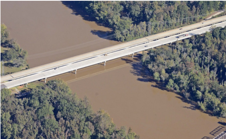
The longest prestressed beam spans in the state of South Carolina in 2017.
