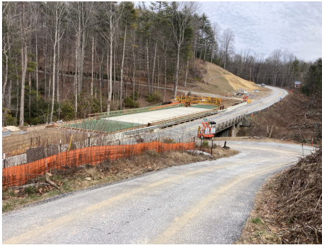
MC444- The bridge deck pour has been completed for phase 1.
