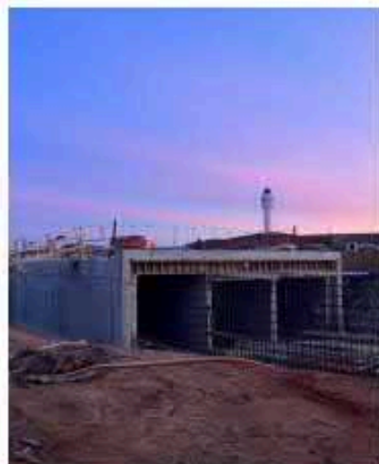
CDIA STOCKPILE IN PROGRESS
